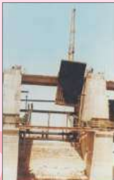
▲ Gate Erection
