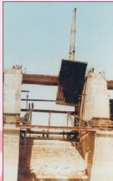
▲ Gate Erection
